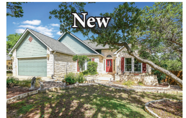
New 3 Springwood Cir. MLS 4826025 New Roof, 3 bdrm + Office 1,586 sq ft, Per- gola, Deck, $419,000 Linda Germain
